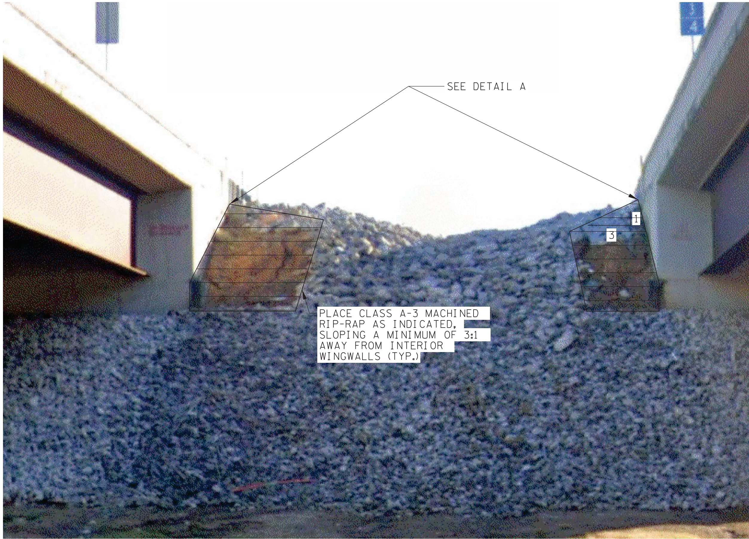
SOUTH ABUTMENT DRAINAGE IMPROVEMENTS (LOOKING BACK STATION)
