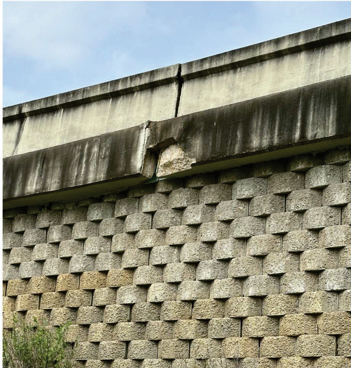
CONCRETE REPAIR AT RETAINING WALL CAP (BRIDGE 24-10269-0123R LOOKING BACK STATION)
